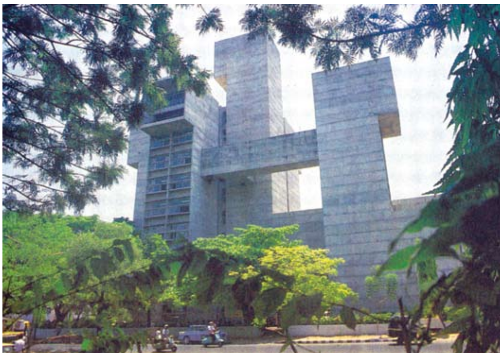
Visvesvaraya Tower, Podium Block, Bangalore
